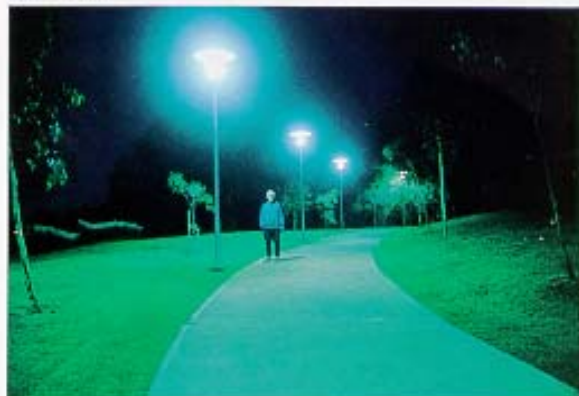
Figure 6. A pedestrian pathway lit to P1 standard by modern luminaires with good glare control and low UWLR, producing high vertical and horizontal illuminances on pedestrians and the pathway.
