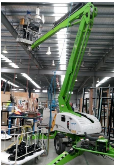
Installation of the new LED high bays and controls
