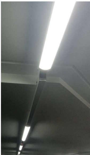
LED batten fittings replacing old T5 fluorescent tubes
